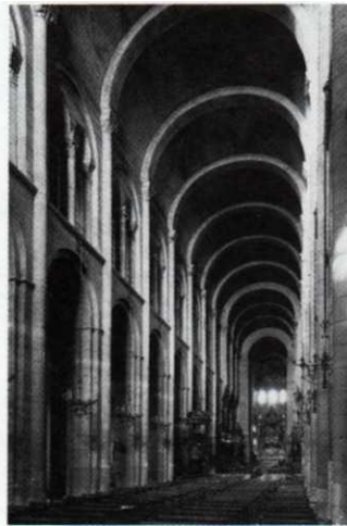
The nave of St. Sernin showing barrel vaults, c. 1080–1120.
