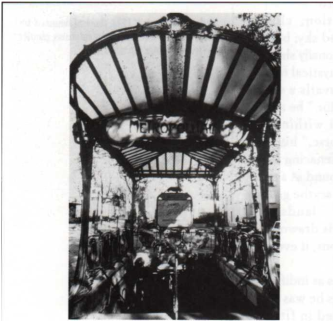
Hector Guimard, Entrance to the Metro, c. 1900, Paris. This wrought-iron entrance to the Paris Metro, or subway, shows the curliag, orgaaic, plantlike style of Art Nouveau
