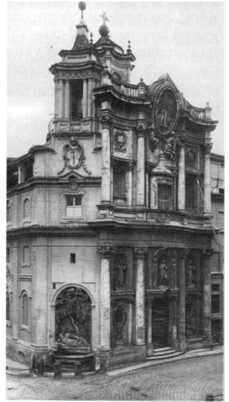
Borromini, facade, San Carlo alle Quattro Fontane, 1665-67, Rome. Borromini's trademark was alternating convex and concave surfaces to create the illusion of movement.
