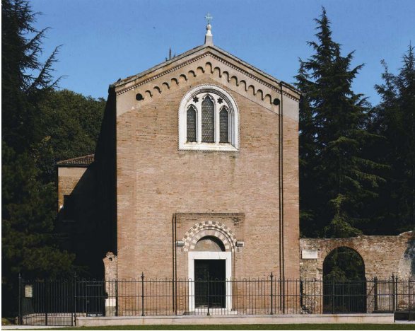
Arena (Scrovegni) Chapel
